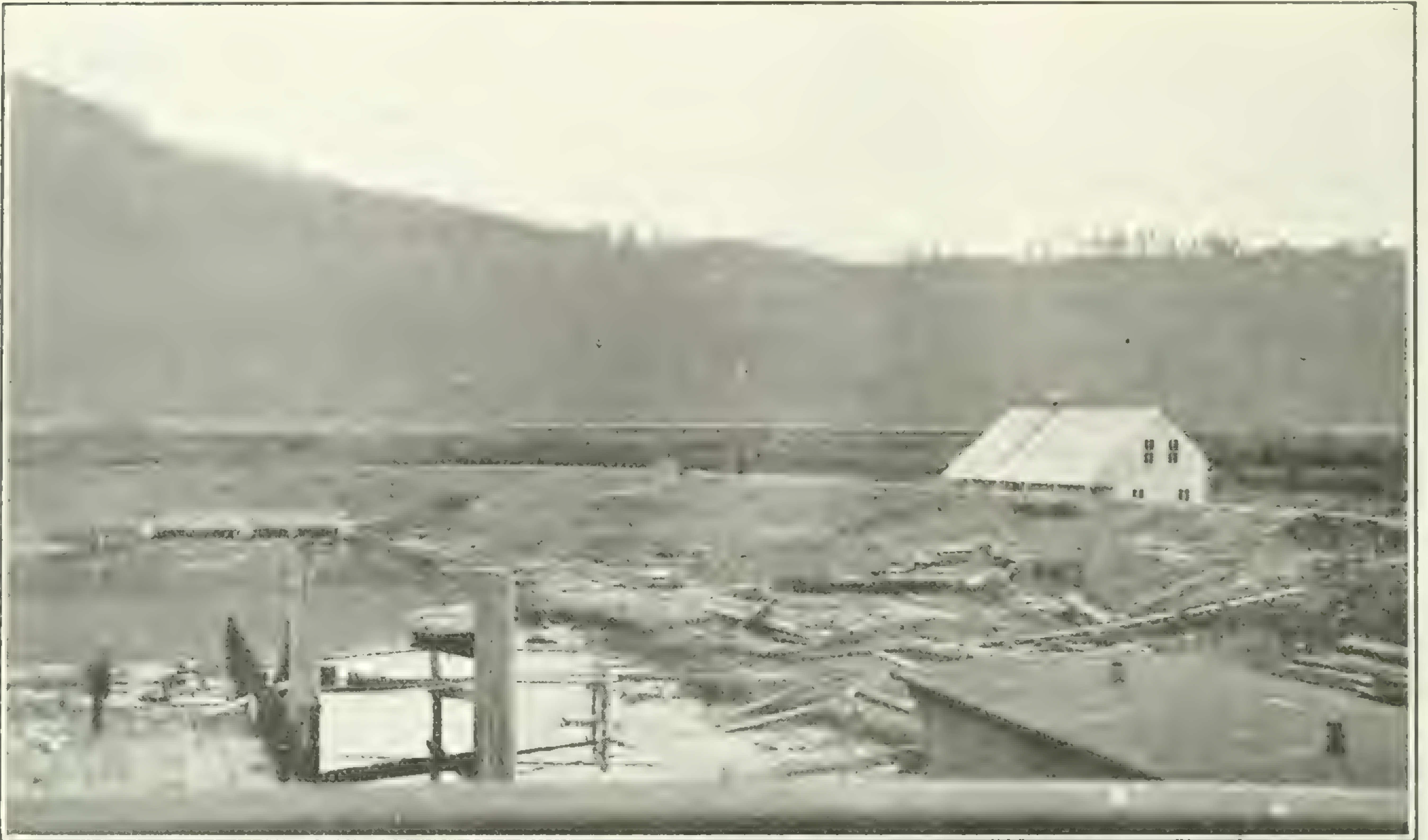
Reclamation-Pitt Meadows Dyke South of Sturgeon Slough.
